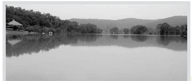
■ Flood levels near Mulla Villa during the June 2007 floods. Photo courtesy of Caroline Maul, Mulla Villa.
